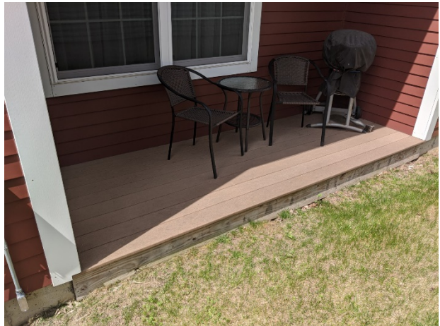
Typical deck at rear of unit
