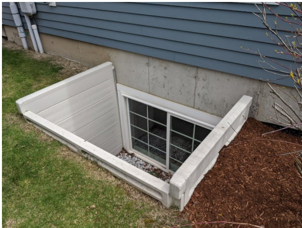
Window well retaining wall overview
