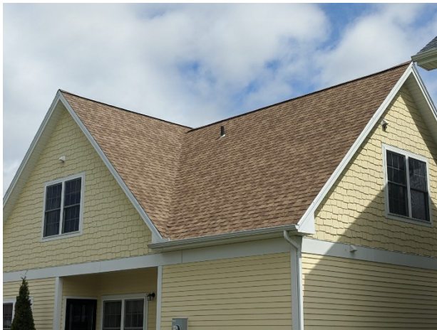
Asphalt shingle roof overview
