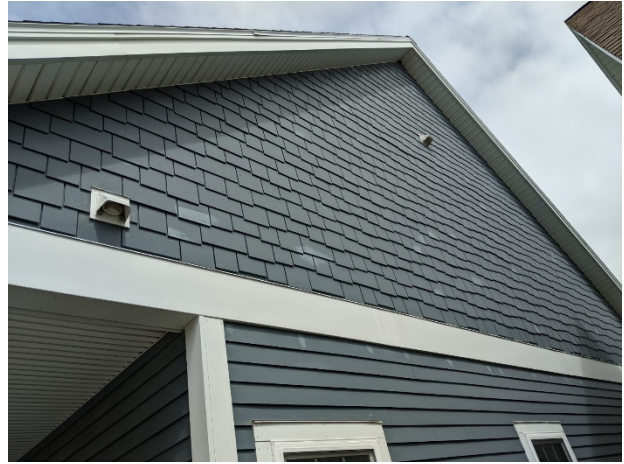
Soffit and fascia at gable
