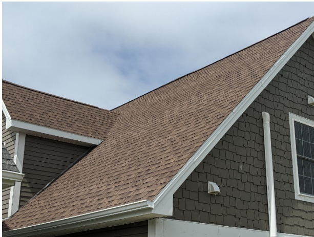
Asphalt shingle roof overview
