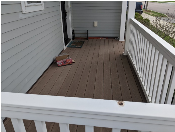
Deck boards at porch
