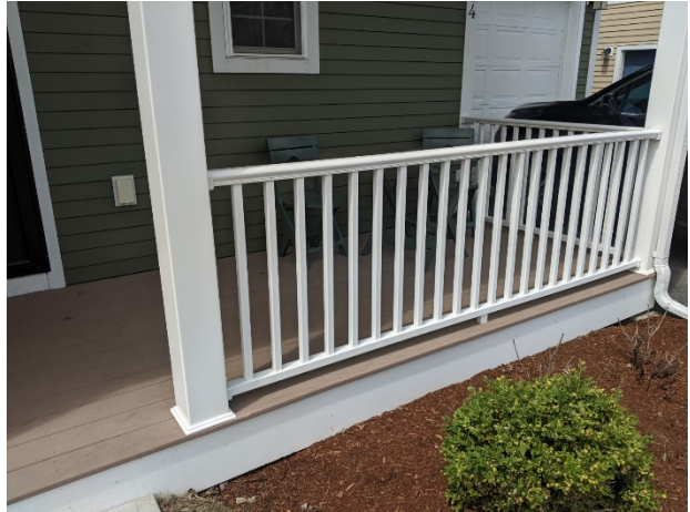
Vinyl railing at porch
