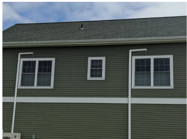
Windows at rear elevation
