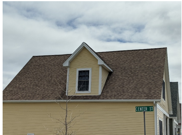
Asphalt shingle roof overview
