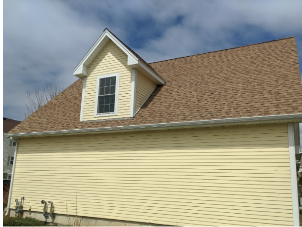
Asphalt shingle roof overview
