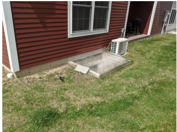
Window well overview with cover
