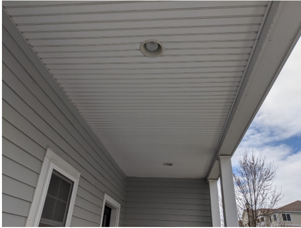
Soffit at porch
