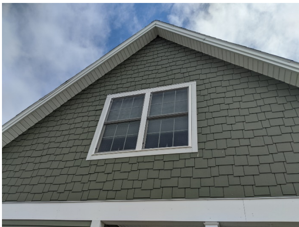
Windows at gable
