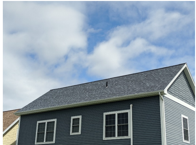
Asphalt shingle roof overview
